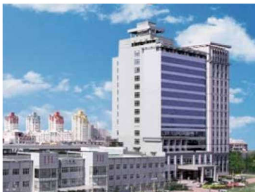
Tianjin Cancer Hospital Chine
