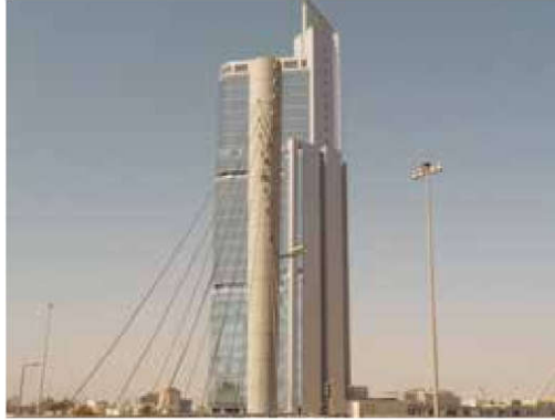
Al Hugayet Tower Offices – 31 floors Kingdom of Saudi Arabia
